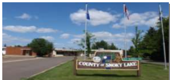
Administration Office located at 4612 McDougall Drive in the Town of Smoky Lake.
