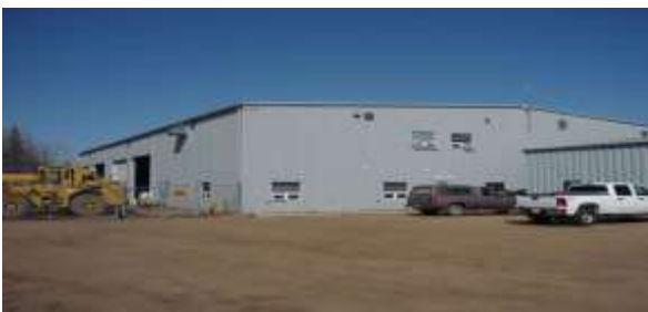
County Public Works Shop located at 5004-50 Street in the Town of Smoky Lake.
