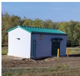
Edwand Booster Station
