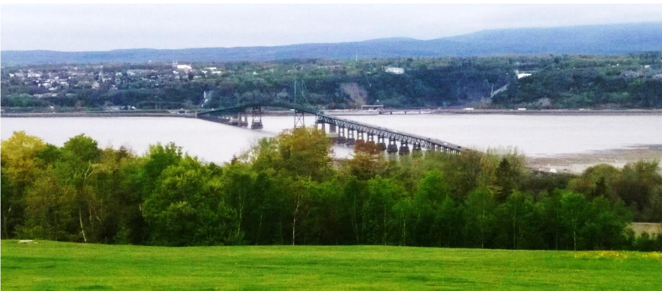
Bridge access across the St. Lawrence River from Quebec to Île d'Orléans, Site Visit May 29, 2019
