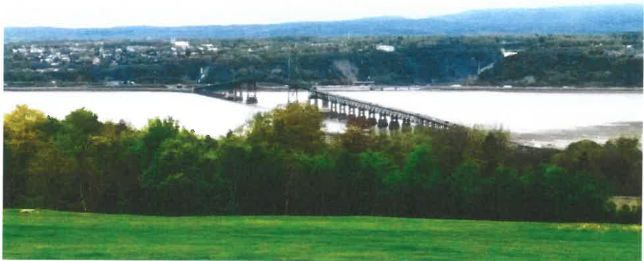
Bridge access across the St. Laurence River from Quebec to Île d'Orléans, Site Visit May 29, 2019
