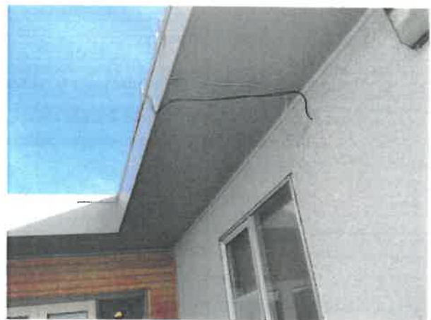
Figure 3-30 Non-vented Soffit
