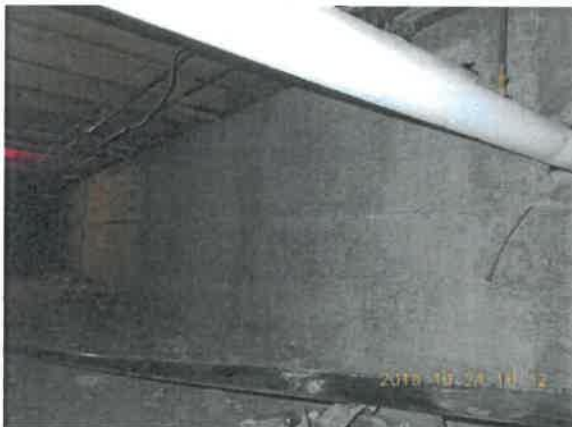
Figure 4-1 Interior Strip Footings Appear to be in Good Condition
