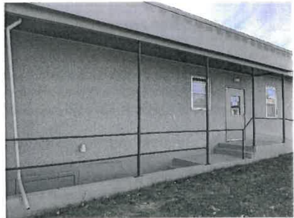
Figure 6-12 Basement Stairwell Lighting
