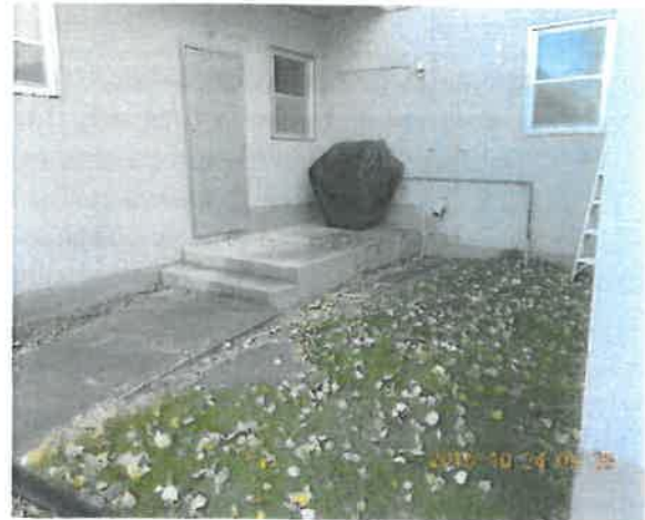
Figure 6-14 Light Broken, Exposed Wiring Above Door
