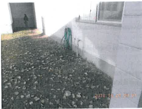
Figure 2-1 Viewing Depression at South Wall of Chambers
