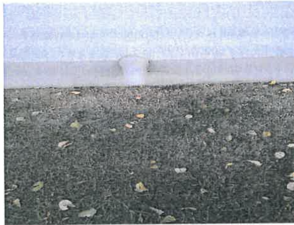
Figure 5-7 Downspouts Close to Foundation
