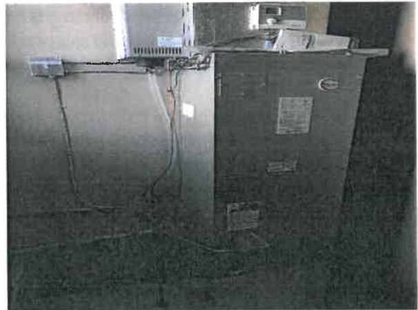
Figure 5-14 Direct Expansion Fan Coil
