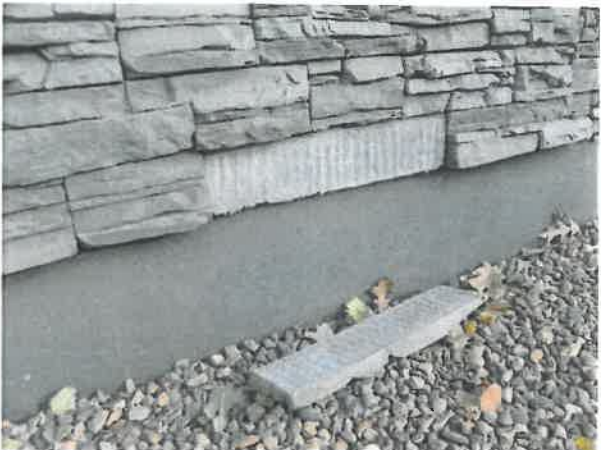
Figure 3-10 Dismounted Stone Veneer
