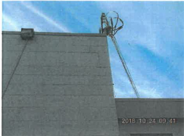
Figure 4-16 Viewing Wide Cracking Through Joints at NW Corner Boiler Room
