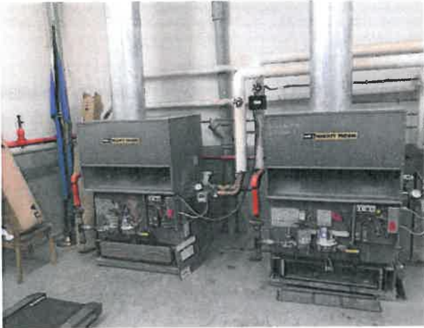
Figure 5-9 Heating Boilers
