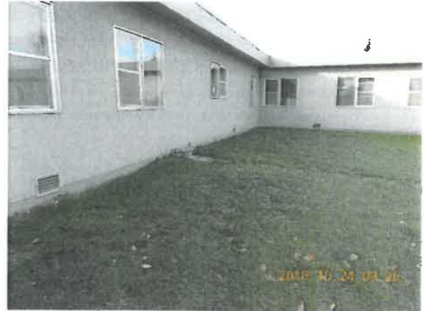
Figure 2-4 Viewing Depression in Grade Along North Wall
