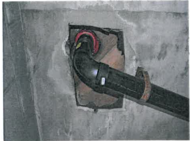
Figure 3-33 Water Stain on Ceiling Around Roof Drain Over Smoke Room
