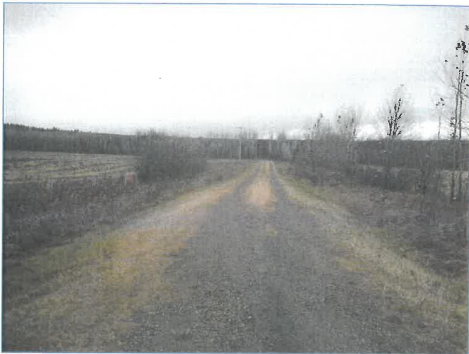
Depicting the trail within the Road Allowance to the north of the Subject Property. Facing north from the north boundary of the Subject Property. The trail within the Road Allowance intersects with the trail (temporary access road) which transects the adjacent parcel of farmland allowing for access to the Subject Property.
