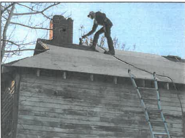
Left: Wilfred Vegelahn nailing the plywood sheathing
