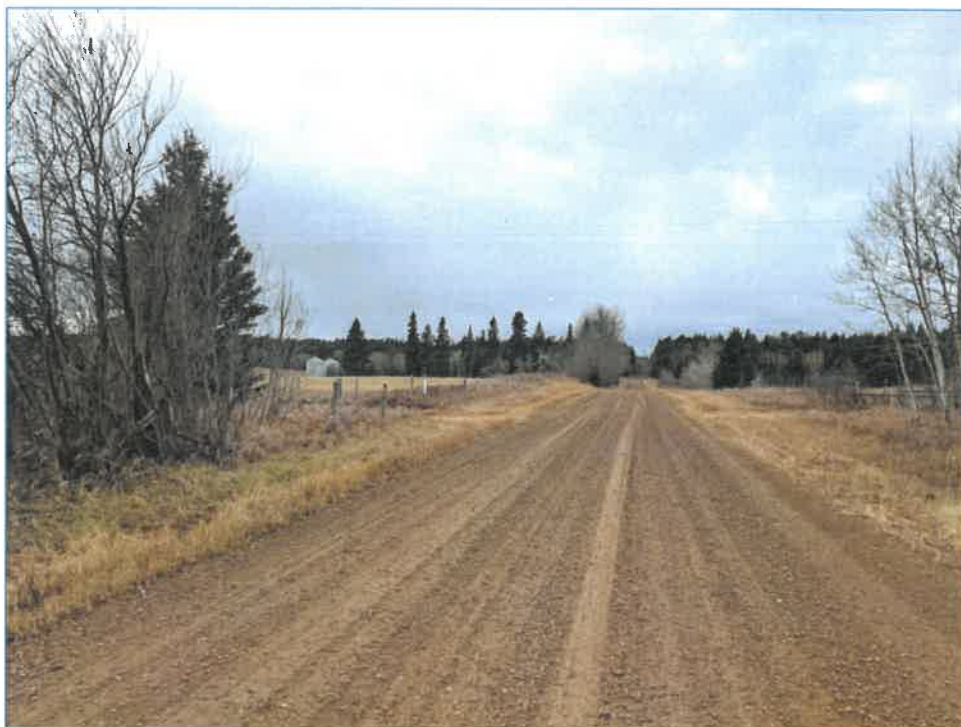
Township Road 590A facing west. The roadway is the closest municipal road to the Subject Property.
