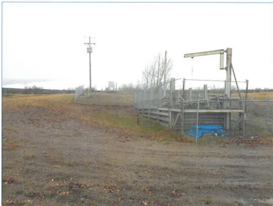
Facing north from near the south boundary of the Subject Property.
