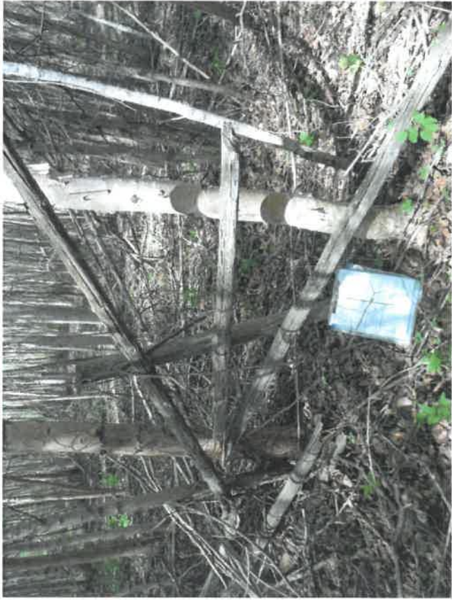
Photo 15: Fencing condition on site
