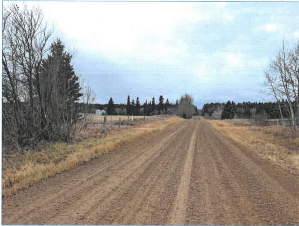
Township Road 590A facing west. The roadway is the closest municipal road to the Subject Property.
