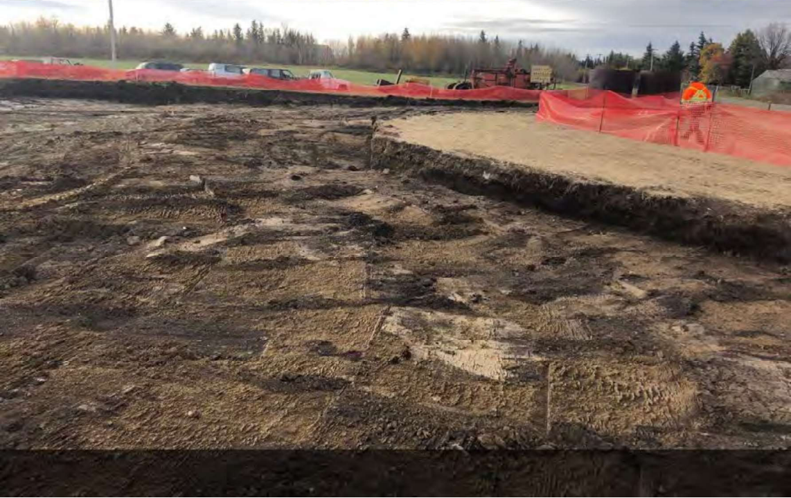
Photograph 5 – Viewing south at excavation (Oct 9, 2020).
