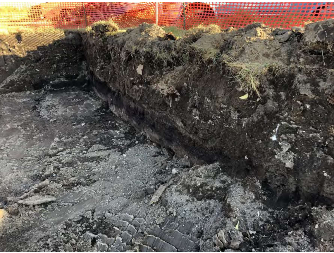
Photograph 6 – Viewing ash material from excavated area (Oct 9, 2020).
