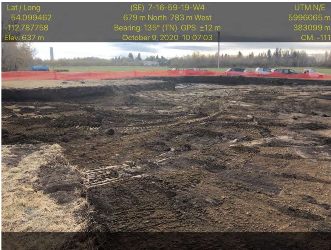
Photograph 4 – Viewing southeast at excavation (Oct 9, 2020).
