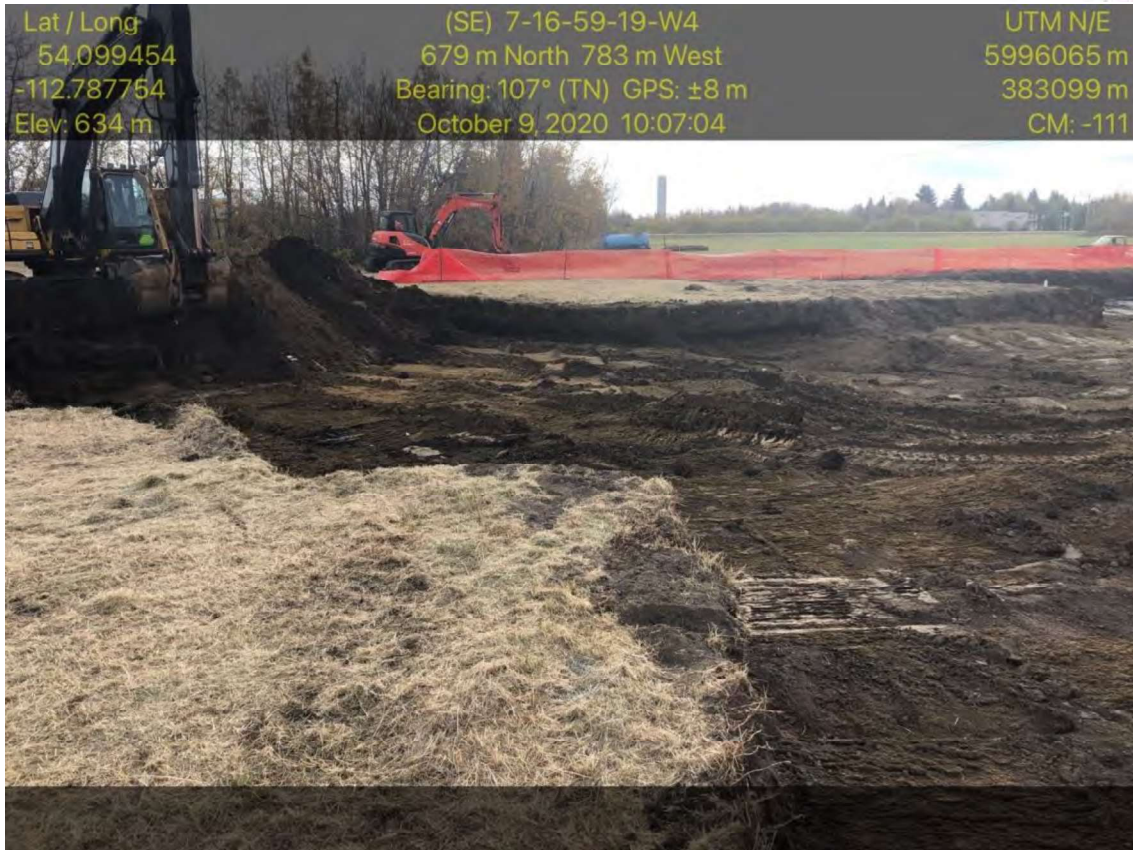
Photograph 3 – Viewing north boundary of excavation (Oct 9, 2020).
