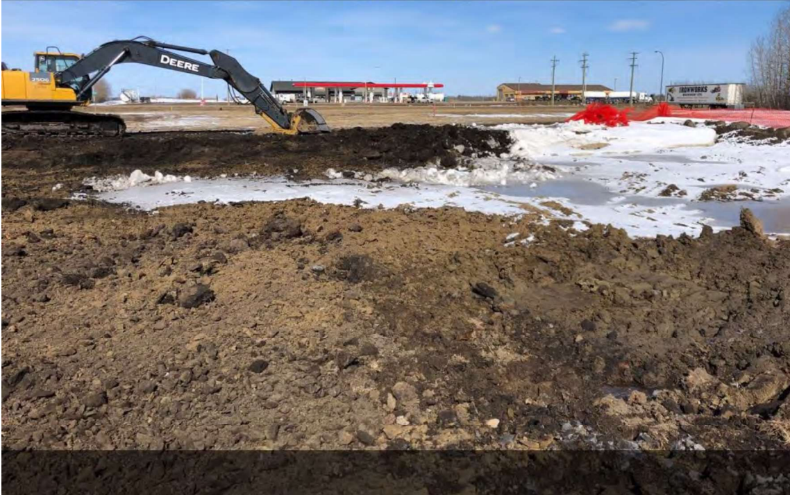
Photograph 10 – Viewing west at additional excavation (March 25, 2021).
