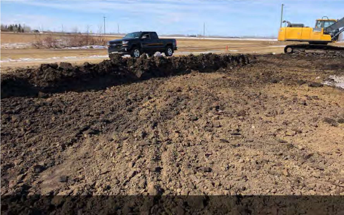
Photograph 9 – Viewing northwest at additional excavation (March 25, 2021).
