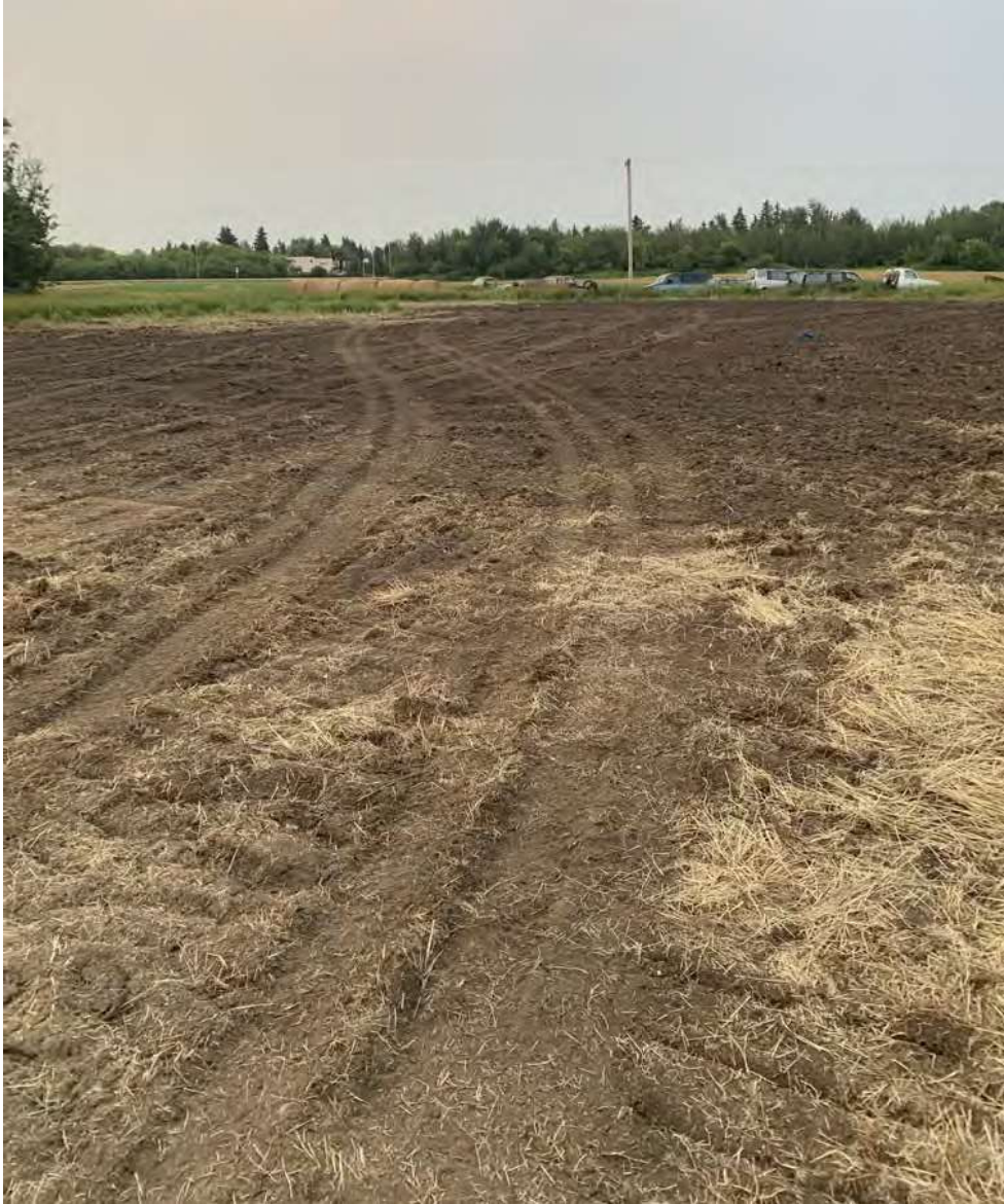
Photograph 11 – Viewing south at backfilled excavation (July 14, 2021).
