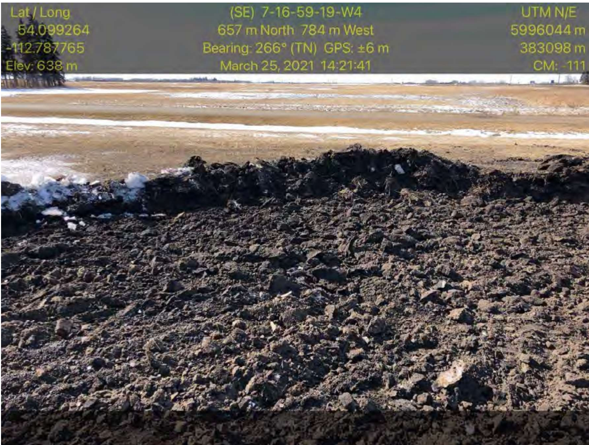
Photograph 8 – Viewing west at additional excavation (March 25, 2021).
