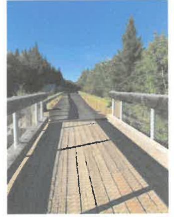
Trestle to pavement
