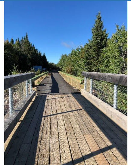
Beaver River Trestle parking lot expansion and paved trail to the trestle. Additional railing was added to stop trail traffic from going up and down the banks which was causing dangerous erosion to the trail surface.
