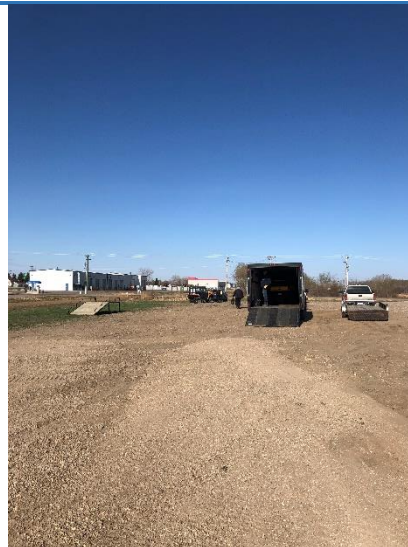
Water line inspection Bonnyville/Cold Lake
