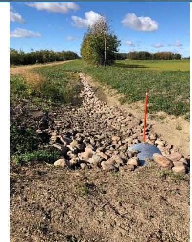
M.D. established drainage for adjacent landowner near Ardmore
