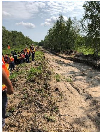
Checking new trenching method.
