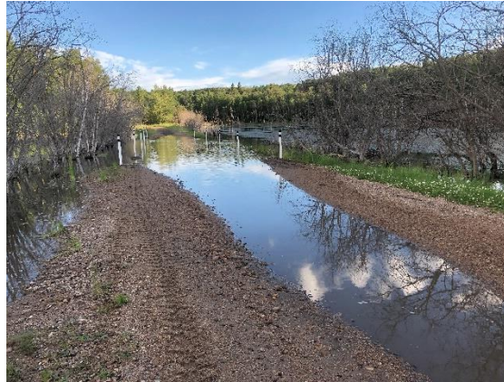
Flooding east of St. Paul. The County installed some delineators to keep users on the trail. Beaver dams were removed, and water receded.
