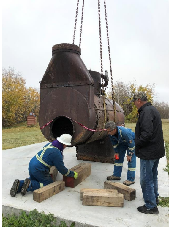
Boiler being delivered and set in place at Abilene Junction. Shelter completed with boiler inside.
