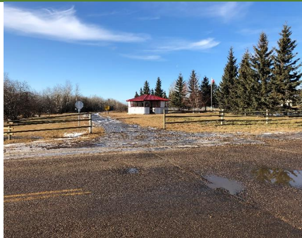
New fencing installed at Ashmont staging area. There was a problem with vehicle traffic driving on the trail. The fencing helped define the staging area and narrowed the trail entrance so it no longer looks like a gravel road.
