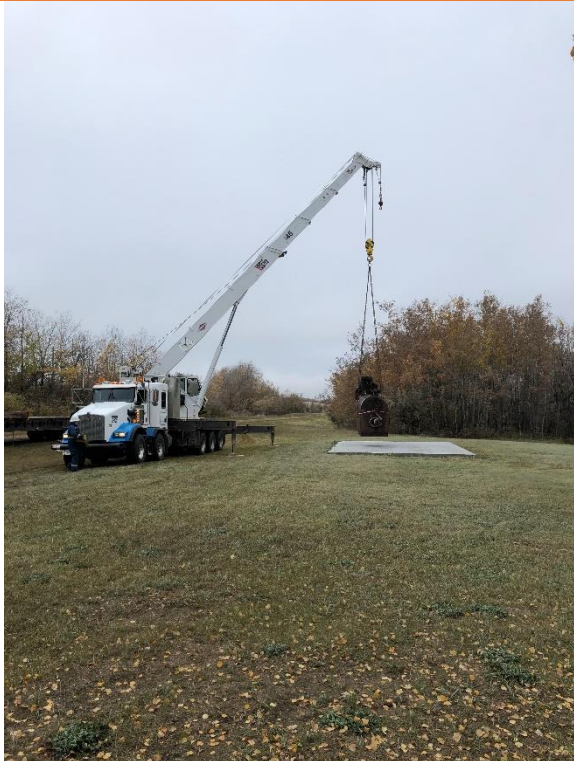
Boiler being delivered and set in place at Abilene Junction. Shelter completed with boiler inside.
