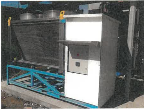
Figure 23 – ORC System (20 kW)
