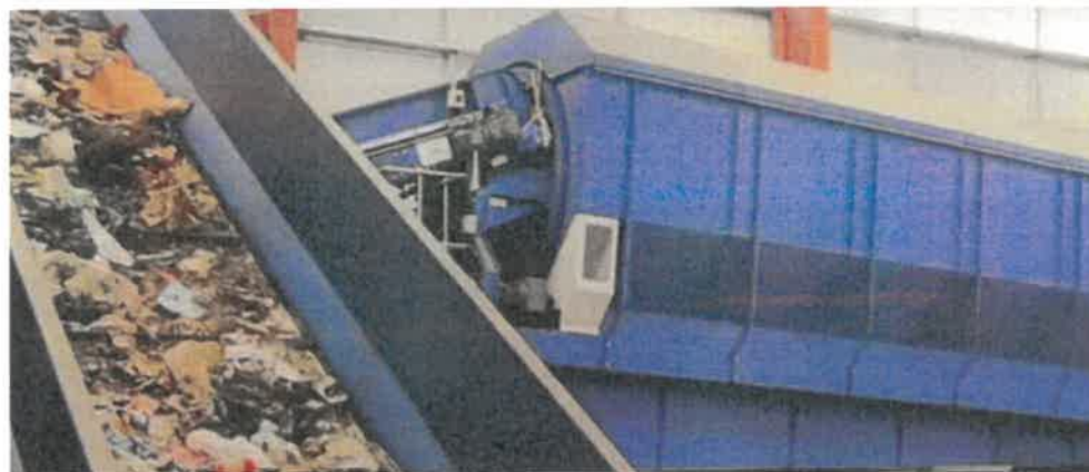
Figure 3: Conveyor to Trommel
