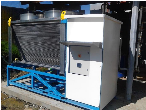
Figure 23 – ORC System (20 kW)
