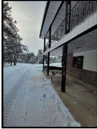
Photo 5 – Residential main house and driveway, facing south.
