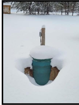
Photo 27 – Entertainment lodge’s septic tank, facing south.
