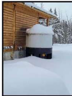
Photo 26 – Entertainment lodge's water tank, facing southwest.
