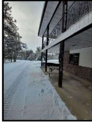
Photo 5 – Residential main house and driveway, facing south.
