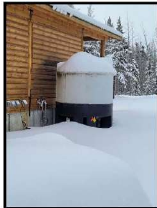
Photo 26 – Entertainment lodge’s water tank, facing southwest.
