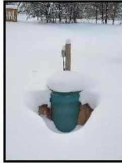
Photo 27 – Entertainment lodge's septic tank, facing south.
