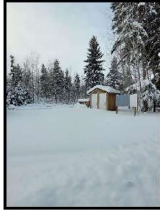
Photo 21 – Campsite washrooms, facing southwest.
