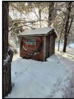
Photo 4 – Storage shed, facing southeast.
