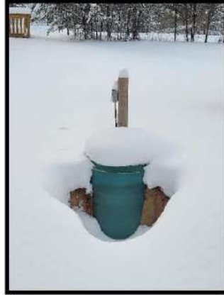
Photo 27 – Entertainment lodge’s septic tank, facing south.
