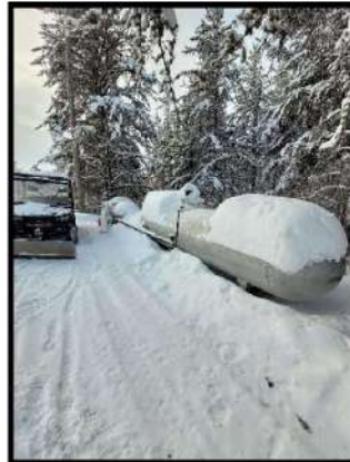
Photo 8 – Two aboveground propane tanks for main household.
