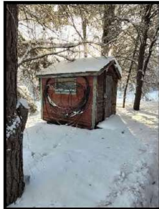
Photo 4 – Storage shed, facing southeast.
