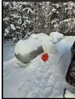
Photo 9 – Empty jerry can adjacent to the two main house aboveground propane tanks.
