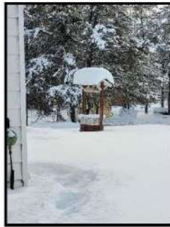
Photo 6 – Main house domestic water well.
