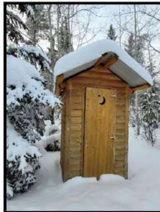
Photo 20 – Campsite outhouse, facing south.
