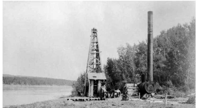
Figure 55. Drilling plant, Victoria Settlement, 1898. Credit: George M. Dawson / Library and Archives Canada / PA-038160.
