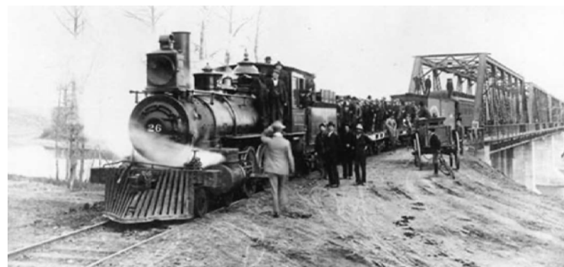
Figure 33. The first train to cross the bridge over the North Saskatchewan River at Edmonton, October 20, 1902. Credit: Glenbow Archives / NA-1244-1.
