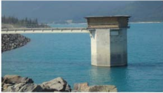
Figure 11. Bighorn Dam intake head gate house
