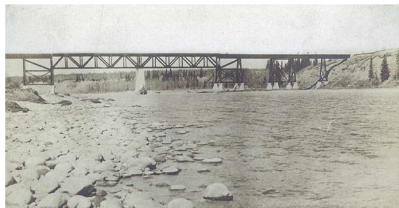
Figure 8. The North Saskatchewan River and bridge, Rocky Mountain House, before 1920. Credit: Peel's Prairie Provinces / Prairie Postcards Collection / PC004774.
