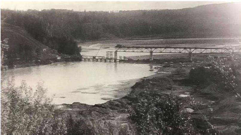
Figure 18. Construction of the bridge over the North Saskatchewan at Drayton Valley, circa 1956. Credit: Drayton Valley Museum.
