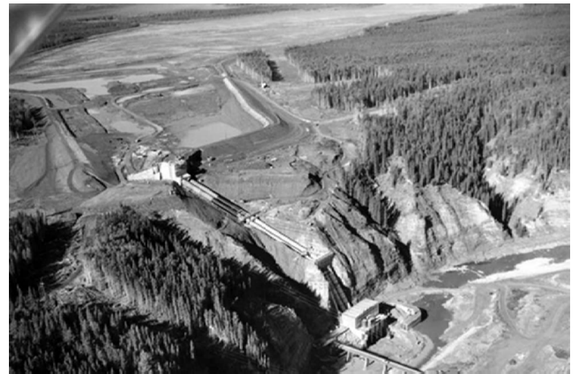
Figure 20. Aerial view of the Brazeau River hydroelectric dam, circa 1960s. Credit: Glenbow Archives / PA-1864-468.
