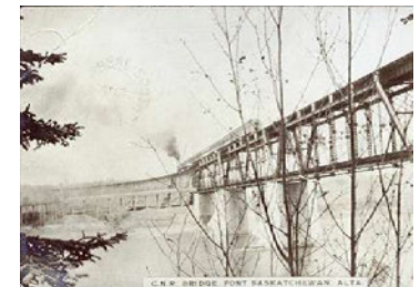
Figure 64. C.N.R. Bridge, Fort Saskatchewan, Alberta, circa 1906. Credit: Peel's Prairie Provinces, Prairie Postcards / PC003653
