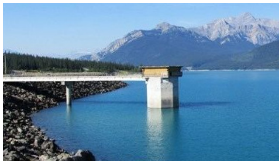
Figure 15. Bighorn Dam intake head gate house
