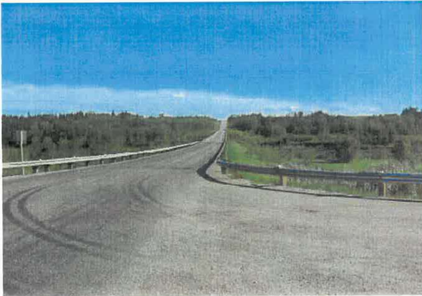
Picture 5 : View South, guardrail.
