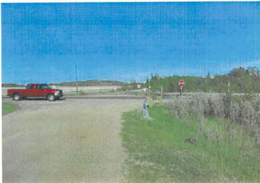
Picture 7 : Looking West at intersection. Guardrail wraps around flare.
