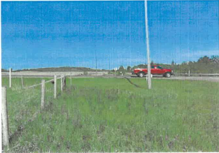
Picture 9 : Powerpoles running East-West
