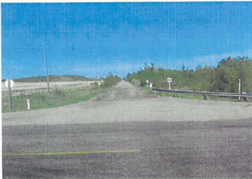
Picture 3 : View of East Leg.
