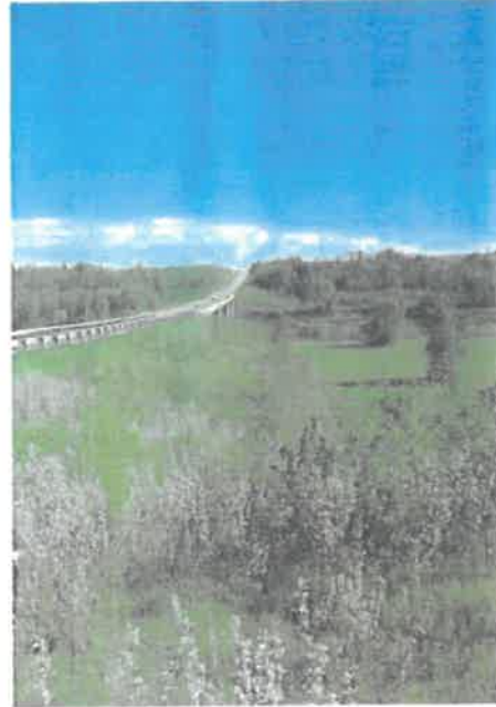
Picture 8 : View South of the slope.
