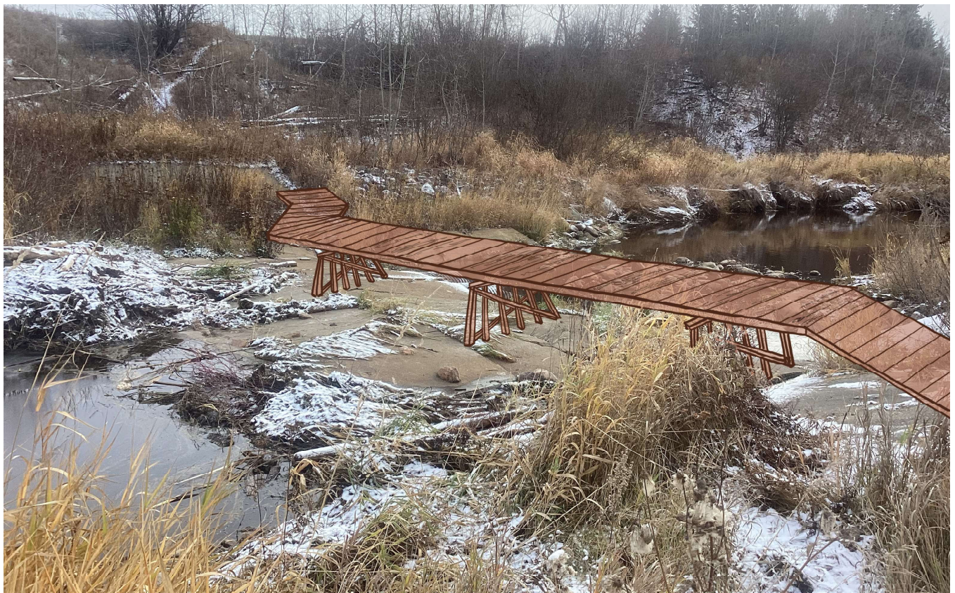
Figure 11. Weir-crossing bridge leading from the existing village nature trails to the fishpond.
