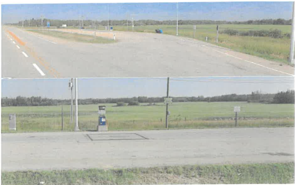
Figure 2. Ground photo of axel weigh scale set up and components in Westlock County near Clyde, AB.
