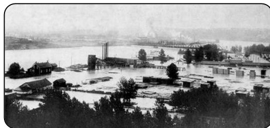
Walterdale Flats John Walter Lumber Mill Bldgs. Image courtesy of the City of Edmonton Archives EA-10-250.
