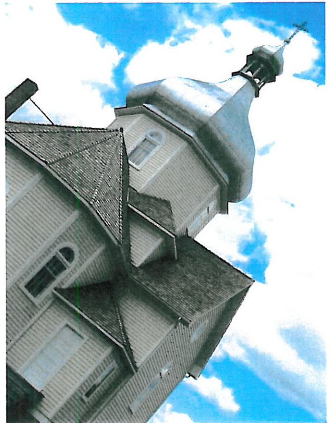
Close up of East Side
