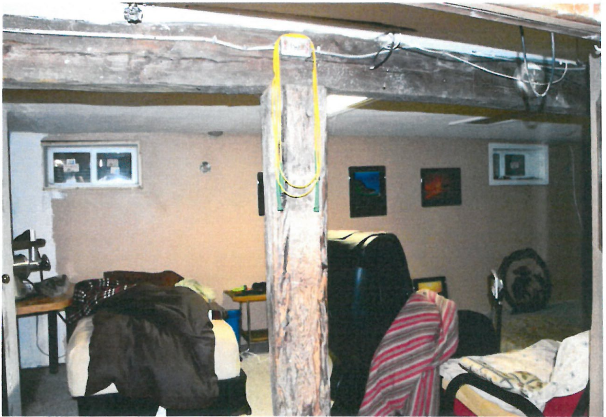
Heavy post and beam construction in the basement
