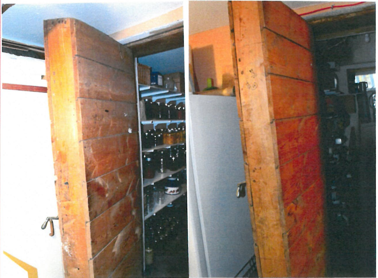
Cold storage door and hardware
