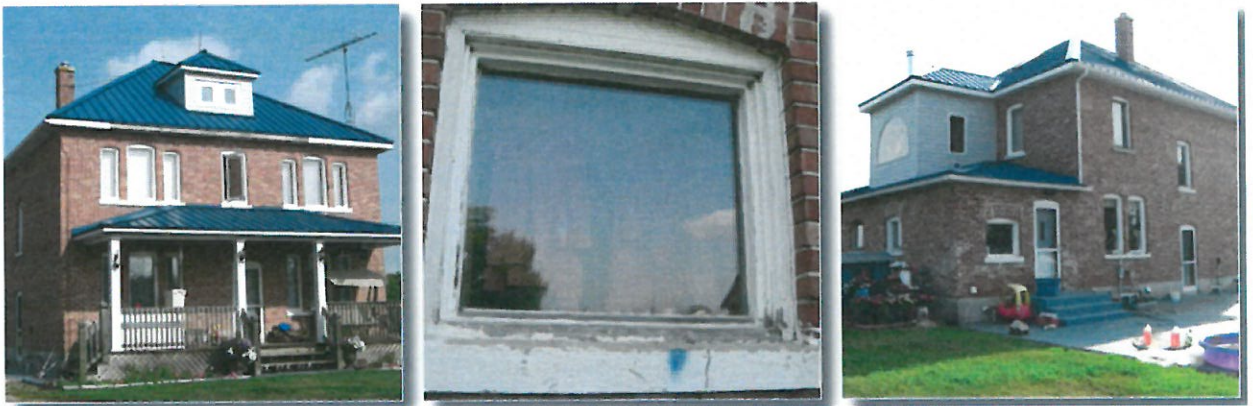
Exterior brick cladding, brick voussior and concrete sill
