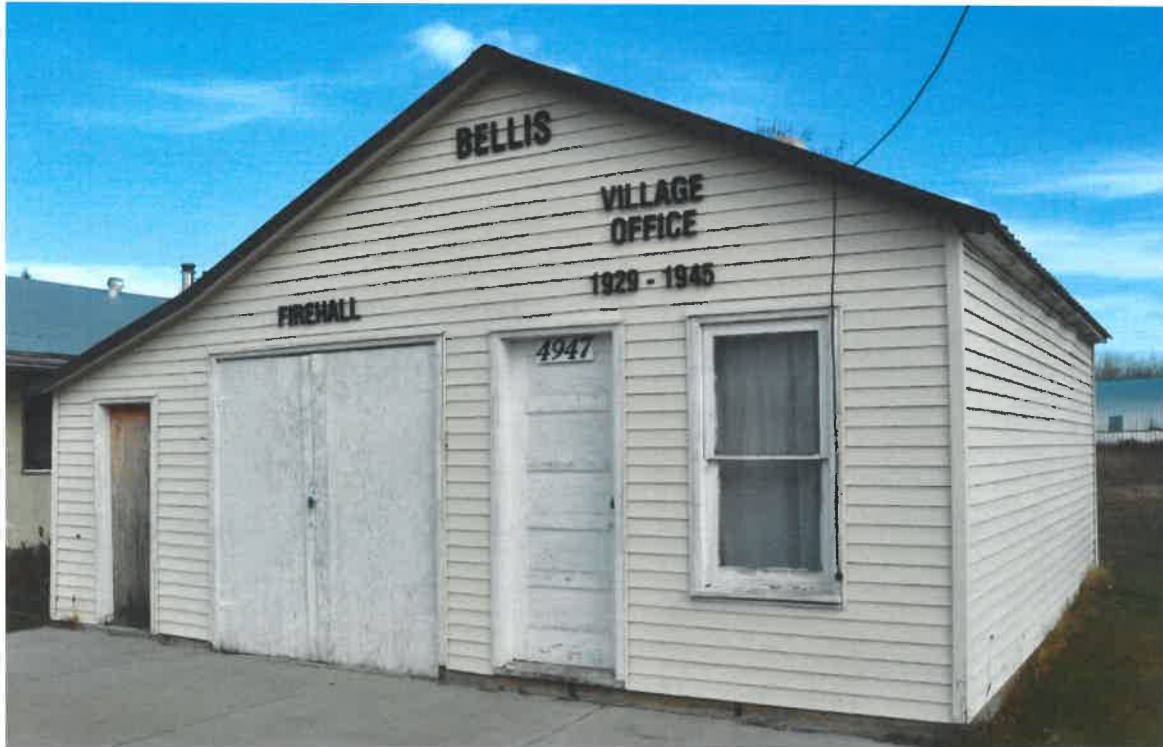
Building Frontage Exterior
