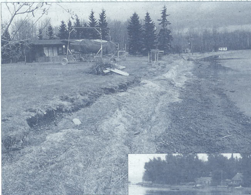
Shoreline Erosion – left. All natural vegetation (aquatic and terrestrial) was removed from the shoreline. Grass was planted to the existing water's edge. In high water years, wave action cut away under the turf, resulting in the loss of feet of property.
