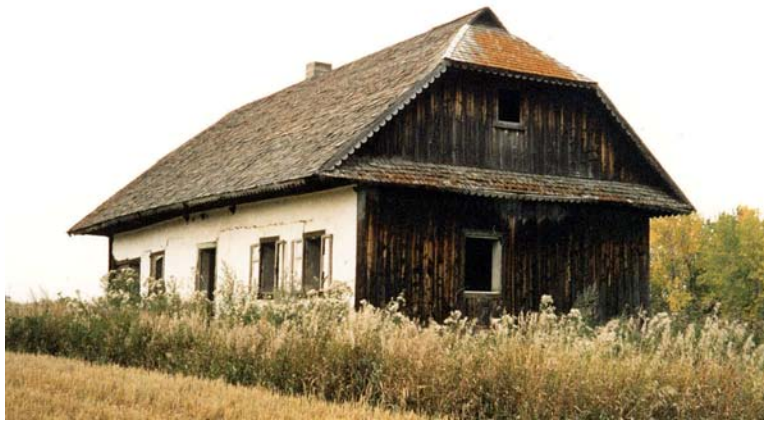
Figure 3.8j: The Goryniuk house constructed in 1925. [Parks/Villeneuve, 2000]
